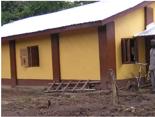
2004 outside Maima School as building work draws to a close
